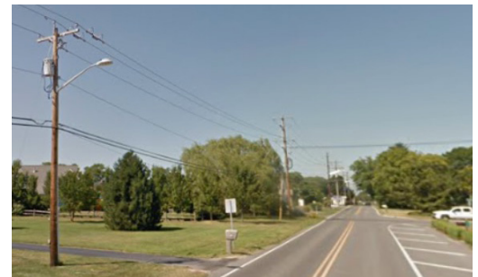
Figure 58 Existing roadway lighting on New Road is limited to the section between 4th Street and Pilottown Road (including approach to 4th Street shown above)
