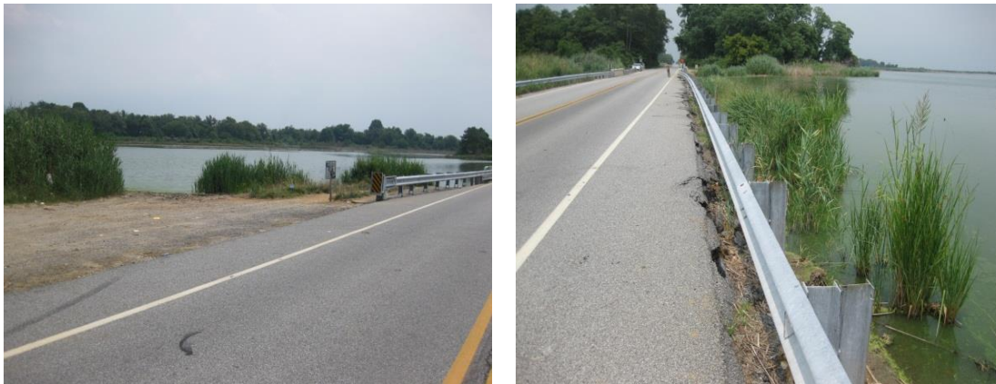
Route 9 North of Port Penn. Note the ‘unofficial pull-off area in the foreground in the picture on the left and the parked vehicle in the background in the picture on the right. Strategically placed pull-off areas would be a benefit to anglers, birders and photographers.
