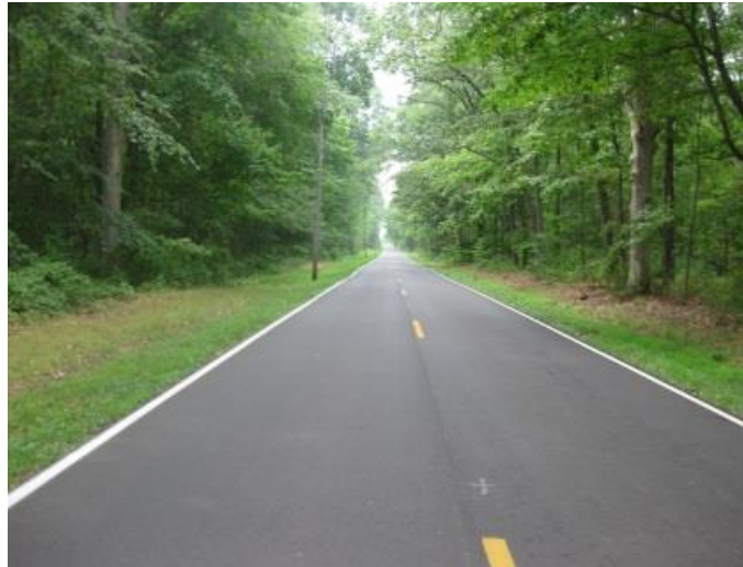
This section of State Route 9 has no shoulders and 10 foot lanes.
