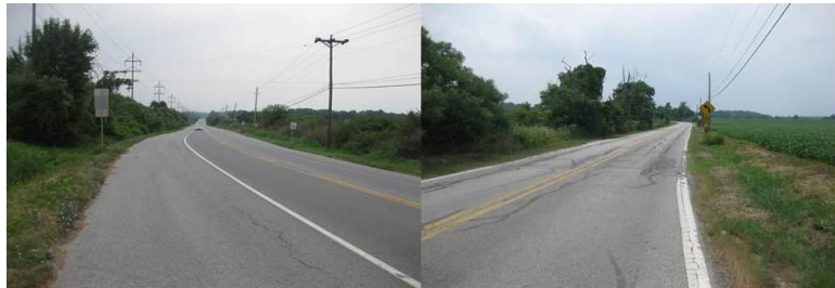
The picture on the left shows State Route 9 in New Castle County which has a shoulder for bicycles to travel separately from the traffic stream. The picture on the right, also in New Castle County, shows a section without bicycle facilities, meaning bicycles and motorized vehicles must share the travel lane.
