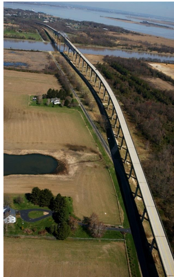
The Reedy Point Bridge is a cantilever truss bridge that carries two lanes of State Route 9 over the C & D Canal. The bridge is 8,432 feet in length. Construction began in 1966 and was completed in 1968. It replaced the last lift bridge over the canal. On a clear day, the views from the bridge are spectacular.
