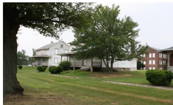
Many buildings, such as the military houses in the photograph, are empty but have the potential to generate revenue and revitalize this important historic site in synergy with the byway vision.
