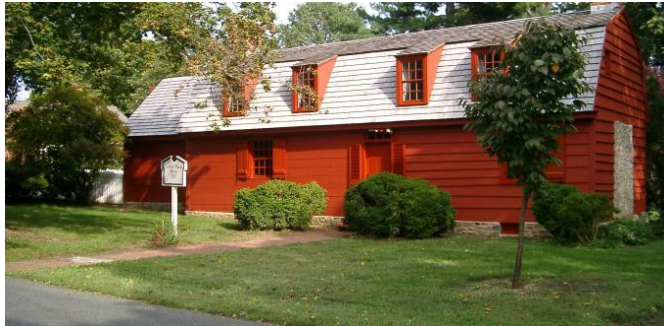
Corbit-Sharp House Photo courtesy of Historic Odessa Foundation
