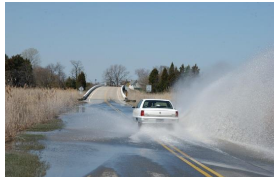
Standing water on Route 9 occurs not only after storms but also after a full or new moon tide.
