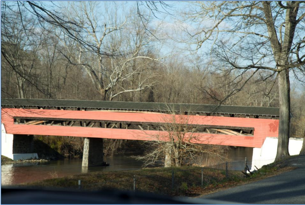
View of Smith Bridge from east side of Brandywine Creek
